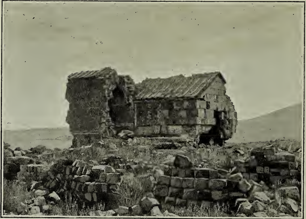
FIG. 81. ANI: BUILDING ON THE CITADEL.
